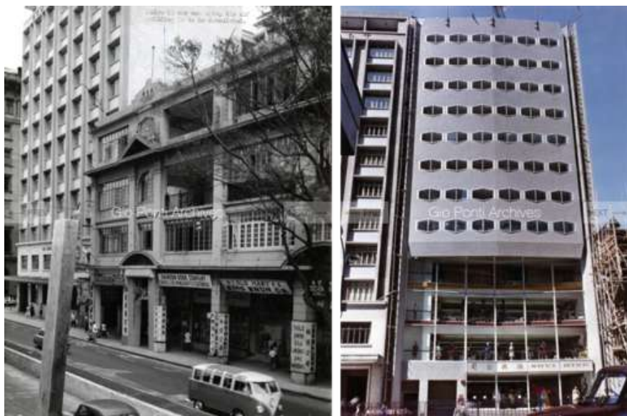
3 | The site on Nathan Road in Tsim Sha Tsui before the construction of Gio Ponti's Shui Hing project in 1963; the Shui Hing project after construction. Source: Gio Ponti Archive, nr. 263EST03, 263EST02.
