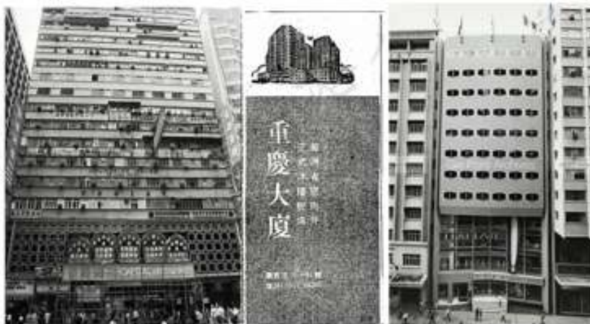
6 | Chungking Mansions (1961) on Nathan Road in Tsim Sha Tsui across from Gio Ponti's Shui Hing project (1963). Source: The Industrial History of Hong Kong Group and Gio Ponti Archives, nr. 263EST05.
